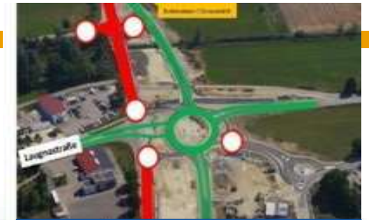
Better infrastructure (Junctions/intersections)
