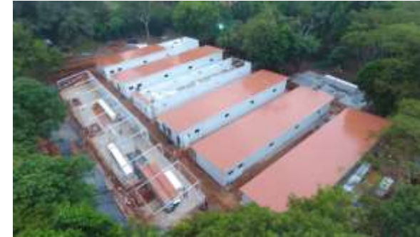
Emergency hospitals under construction
