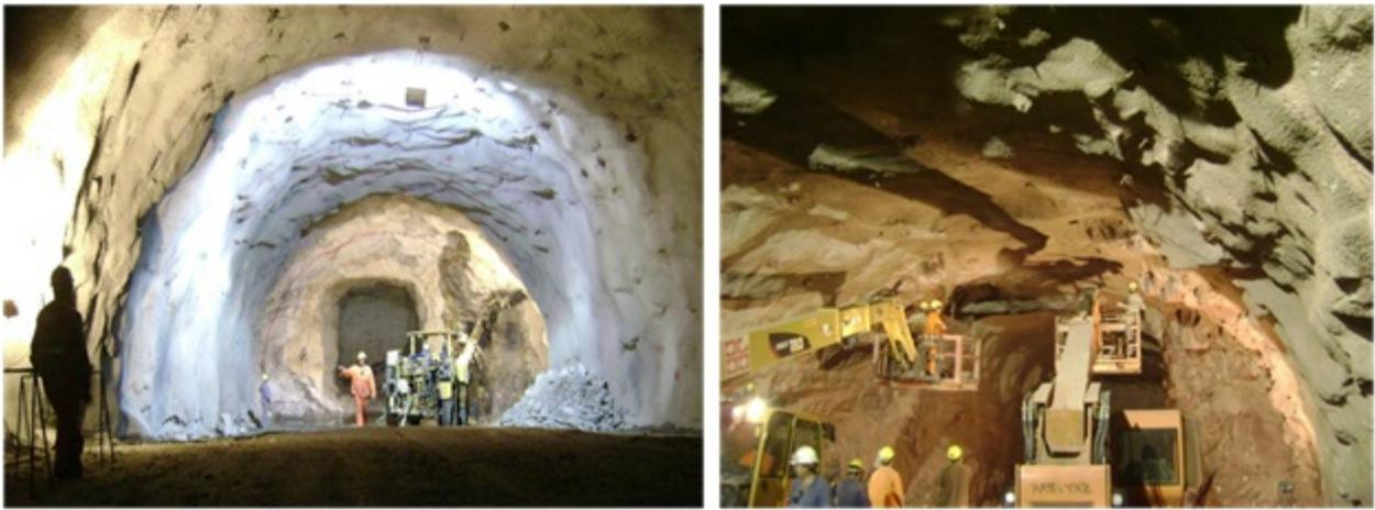
Most tunnels were excavated in formations of poor and very poor rock quality (RMR), with drill and blast methods, where a wide combination of shotcrete reinforced with steel fibres, steel rock bolts and steel ribs was used. The extremely dry climate of the area helps to avoid expensive waterproofing systems.
