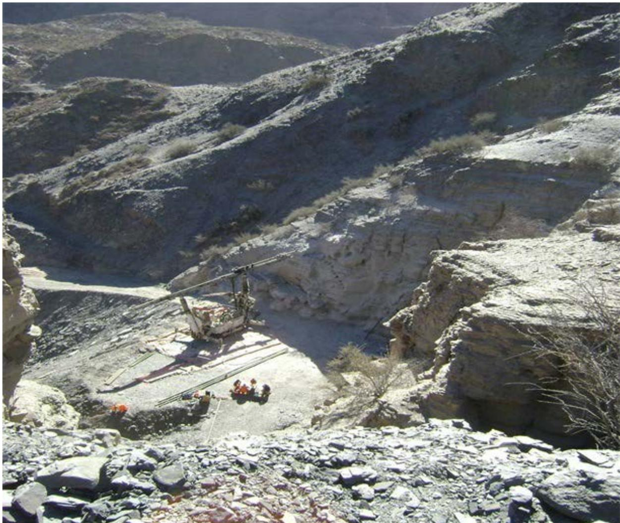
Installing grouted steel pipes at a tunnel portal for pre support of initial excavation rounds.
