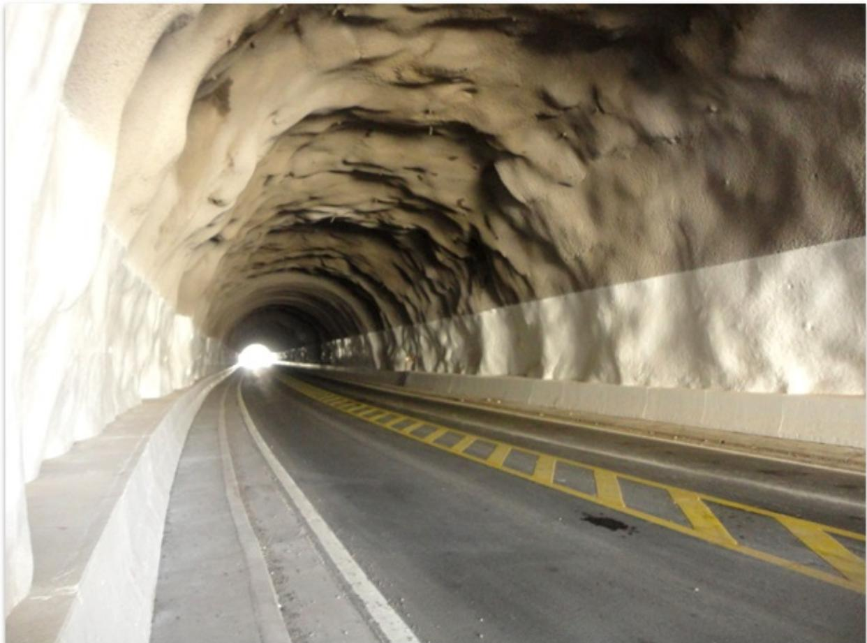
The bidirectional tunnels have two lanes 3,50m wide, a 1,00m central median, two 0,90m sidewalks and New Jersey barriers immersed in the tunnel walls. No lighting was initially provided, as there was no electricity in the area. A recently built transmission line, made possible by the existence of the road, will be used provide energy for tunnel lighting.
